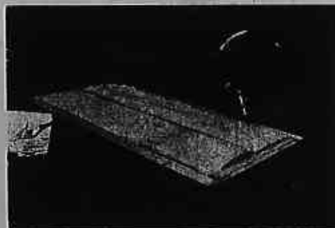
1 Wall panels are glued sandwich of plywood and fir framing with a filler of foil-faced fiberglass insulation.
